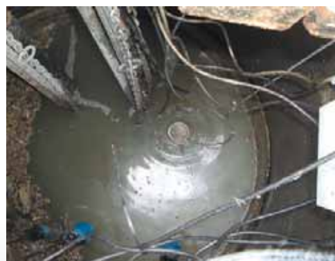
After 14 days of GES treatment: grease cap is radically reduced
